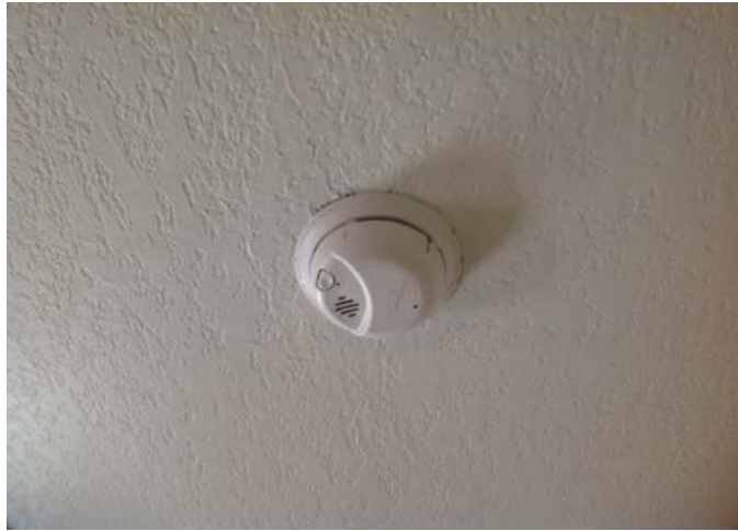
New Smoke Detector
