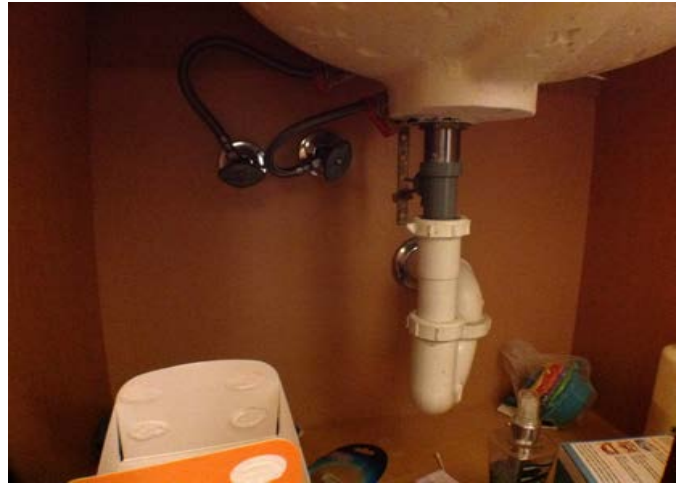
Cabinet Under Sink
