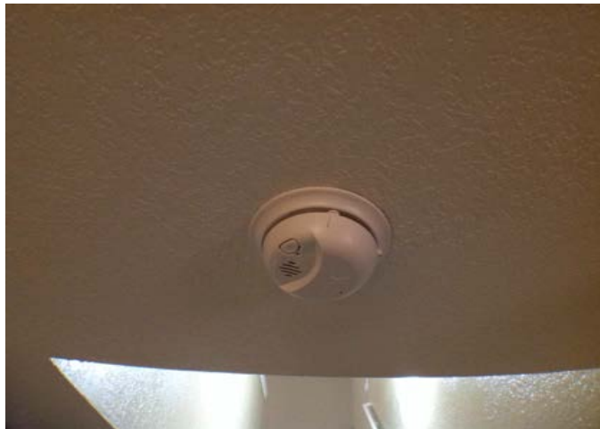
New Smoke Detector
