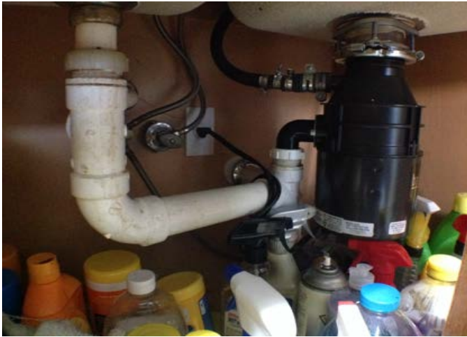
Cabinet Under Sink
