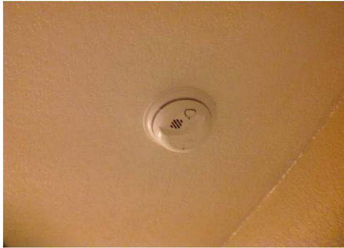
New Smoke Detector
