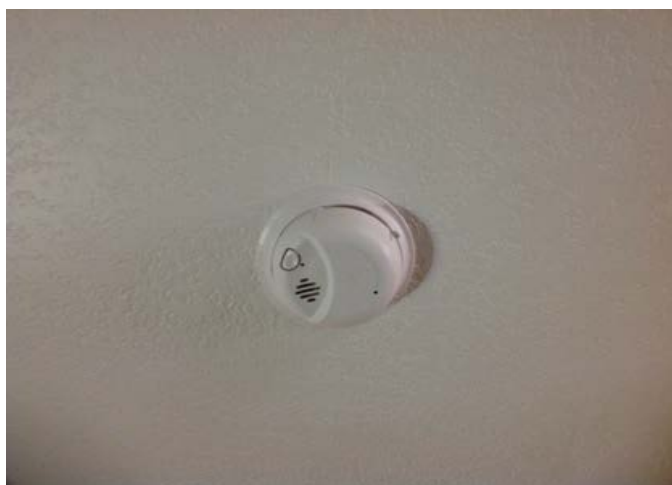
New Smoke Detector
