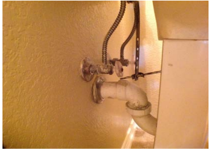
Cabinet Under Sink
