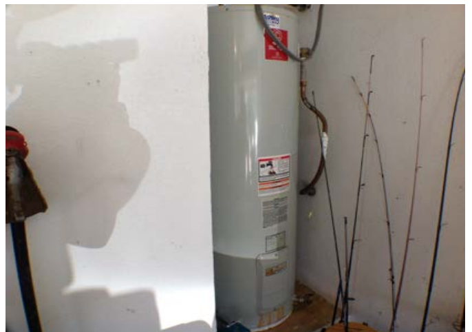
Water Heater(Gas or Electric)
