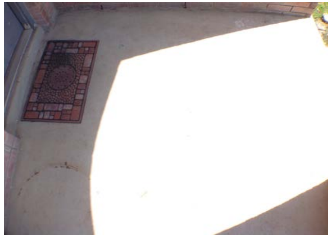
Front Porch Patio
