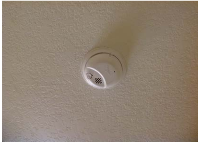
New Smoke Detector
