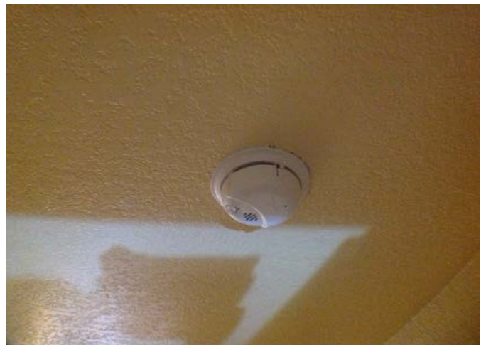
New Smoke Detector
