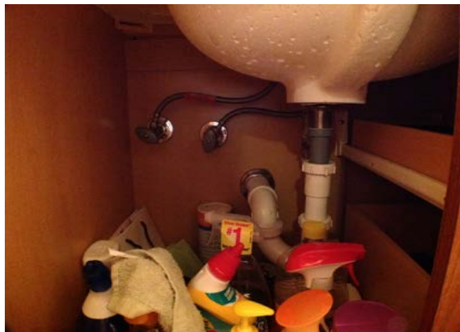
Cabinet Under Sink
